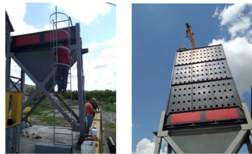
Fig. 7. Installation of the column type grain dryer with the capacity of 5 t/h
